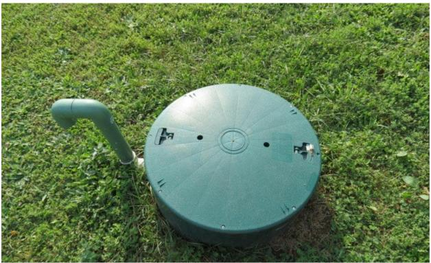
Occasionally tanks may have goosenecks to vent the gasses by the septic tank, which will allow gasses to escape naturally from the tank.
